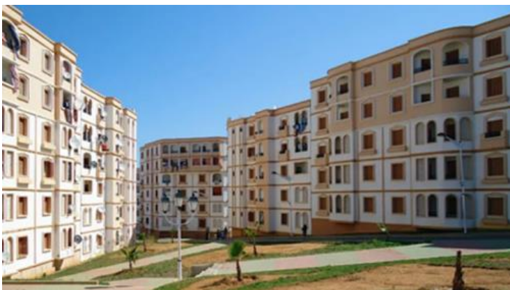
Fig 2– New Residential Buildings for Relocated Residents
